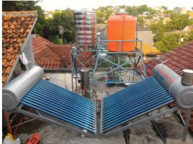
**Gambar 4.** Hasil pembuatan mekanis sistem *indirect evacuated tube solar water heater*
