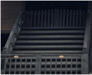
Figure 9. Stairs of Bagas Godang
